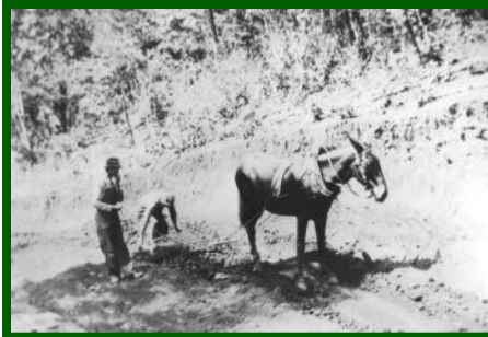
Grading the road to the top of Black Rock Mountain was done by men and mules, 1930s.
