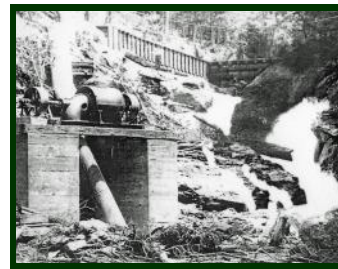
Tom Roane's Power Plant on Stekoa Creek south of Clayton, circa 1915
