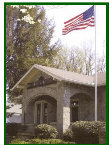
Contemporary photo of the Rock House, which was built in 1935.
