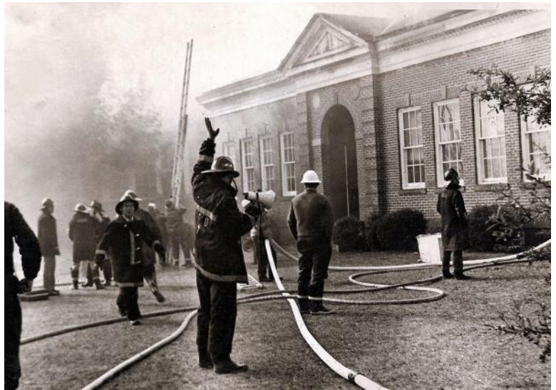
In 1974, the Rabun County High School principal, Frank Snyder, stated that the risk of fire at the 1929 school building was "no joke". He also stated that the school did not have a legitimate occupancy certificate. On Sunday, March 2, 1975, the old high school caught fire, and many of the old buildings were lost. A new school building was under construction at the time, but it was a year before students were able to occupy it.
