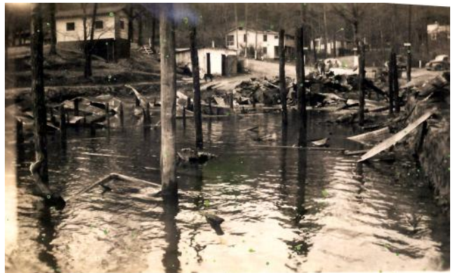
In December of 1951, a blaze completely destroyed the Rabun Boathouse at Lakemont along with boats, motors, equipment and tools.
