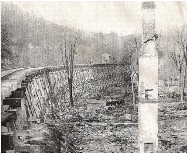
A fire in a mechanic's garage sparked a conflagration that burned the resort town of Tallulah Falls to the ground on a windy December night in 1921. The village had no fire department, and the fire burned out of control.
